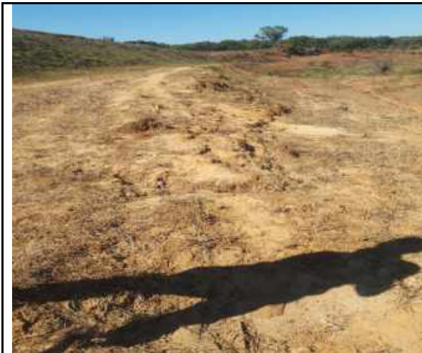
Ant-hills on the downstream slope berm
