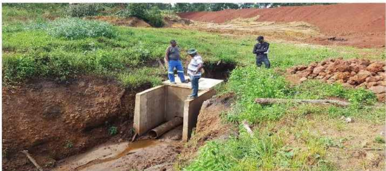
Plate 26: Inspection & Valve Chamber for Irrigation Pipe (COWI Report 2018)
