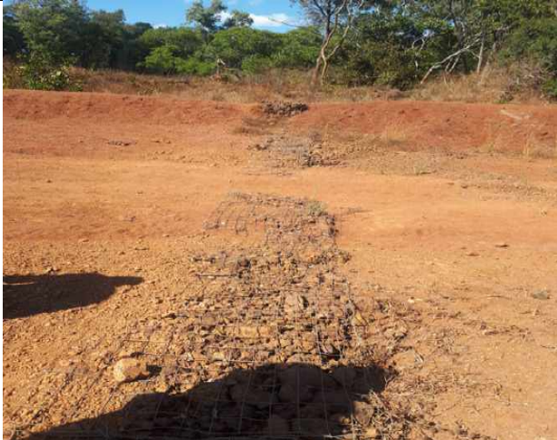
Damaged Gabion Cill due to human and animal tracking
