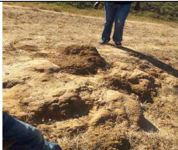
Ant-hill on the downstream slope
