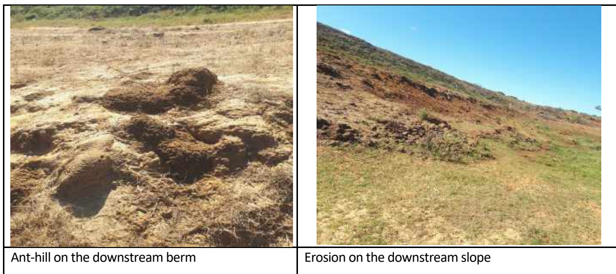
Plate 13: Pictures showing status of downstream slopes
