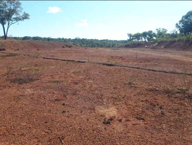
Damaged Gabion Cill due to human and animal tracking
