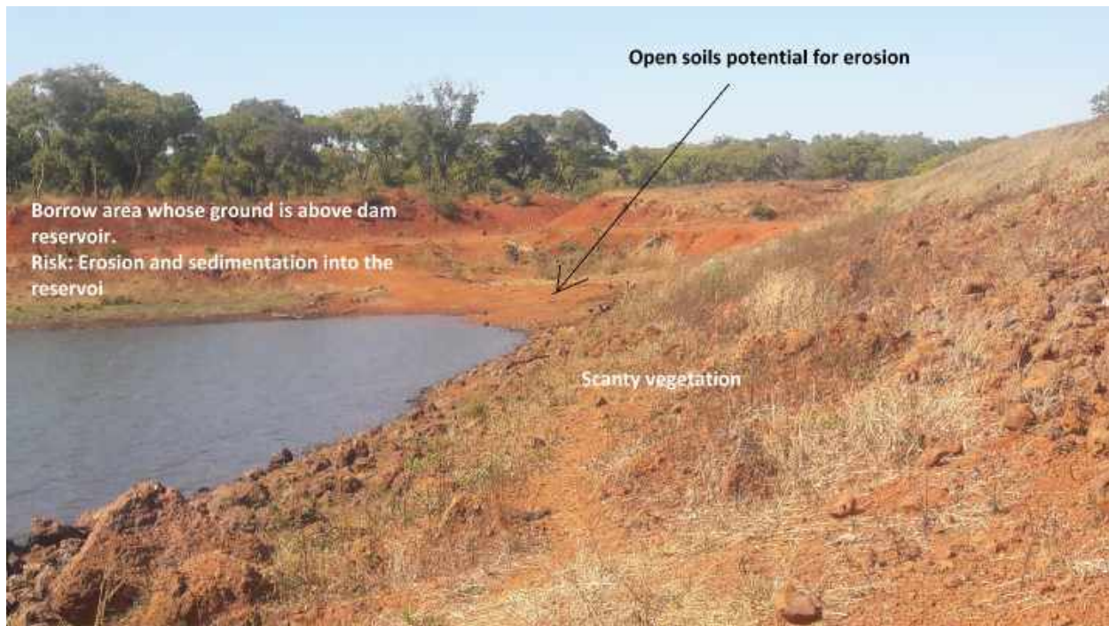
Plate 20: Degraded areas and embankment needing revegetation.
