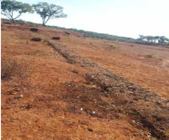
Damaged gabion cill along the spillway return due to human and animal tracking
