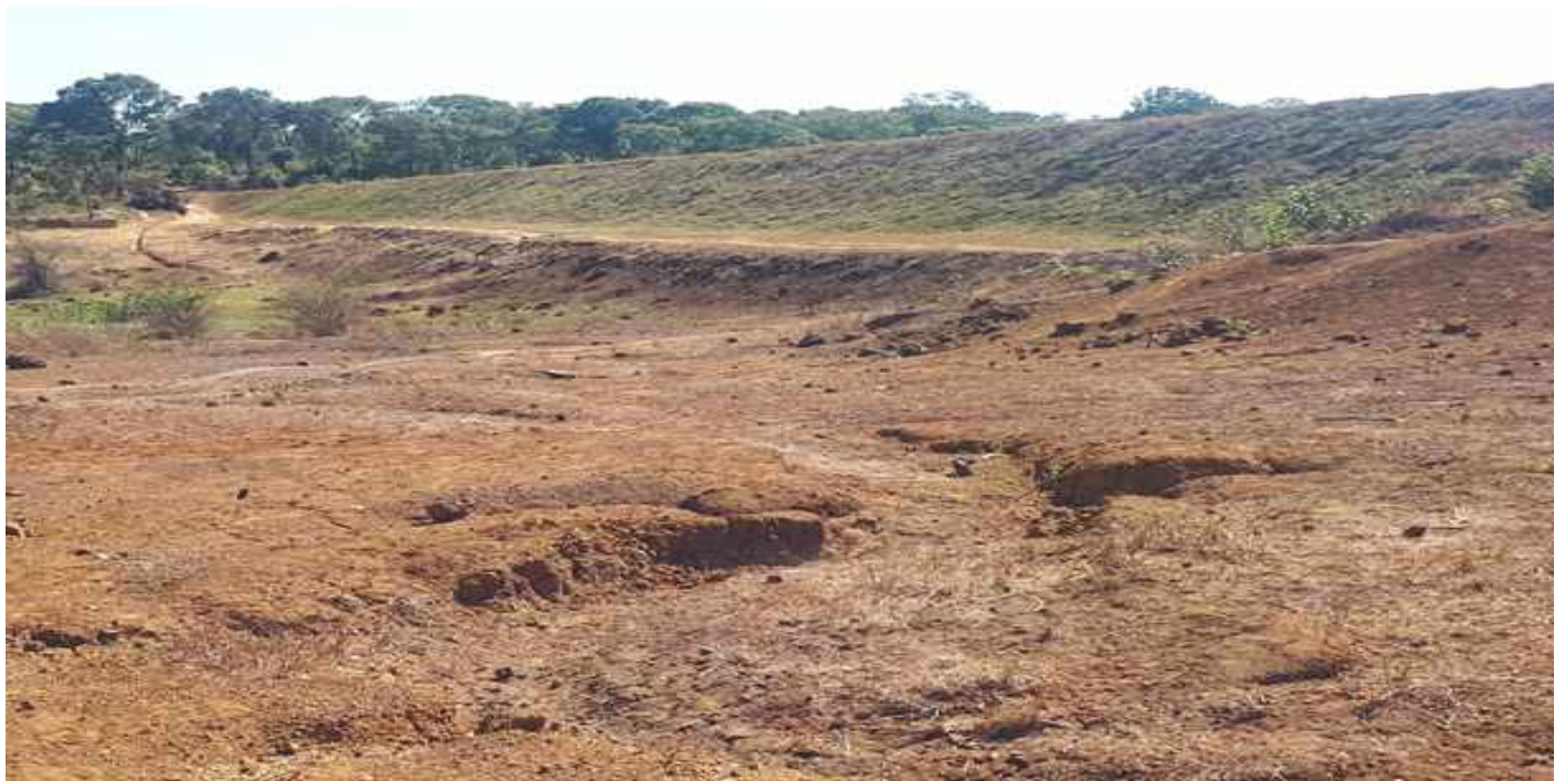
Plate 7: - Embankment Downstream Slope with Berm
