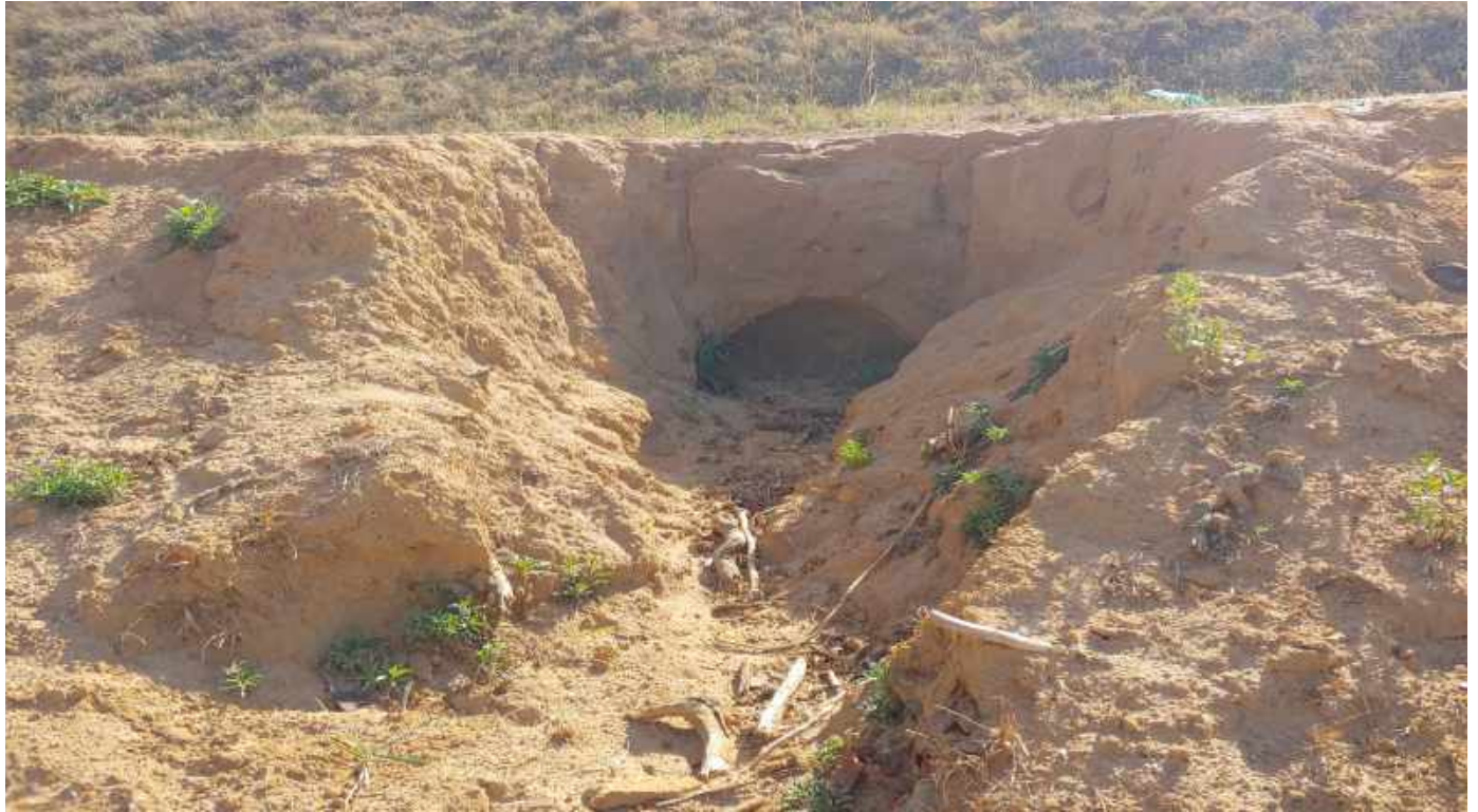
Plate 8: Right Bank Erosion of Suspect Construction Material
