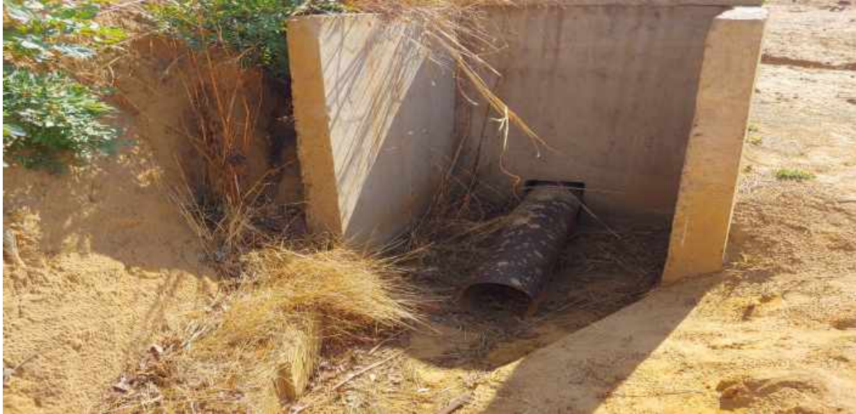
Plate 25: Low Flow Pipe Outlet Valve Chamber
