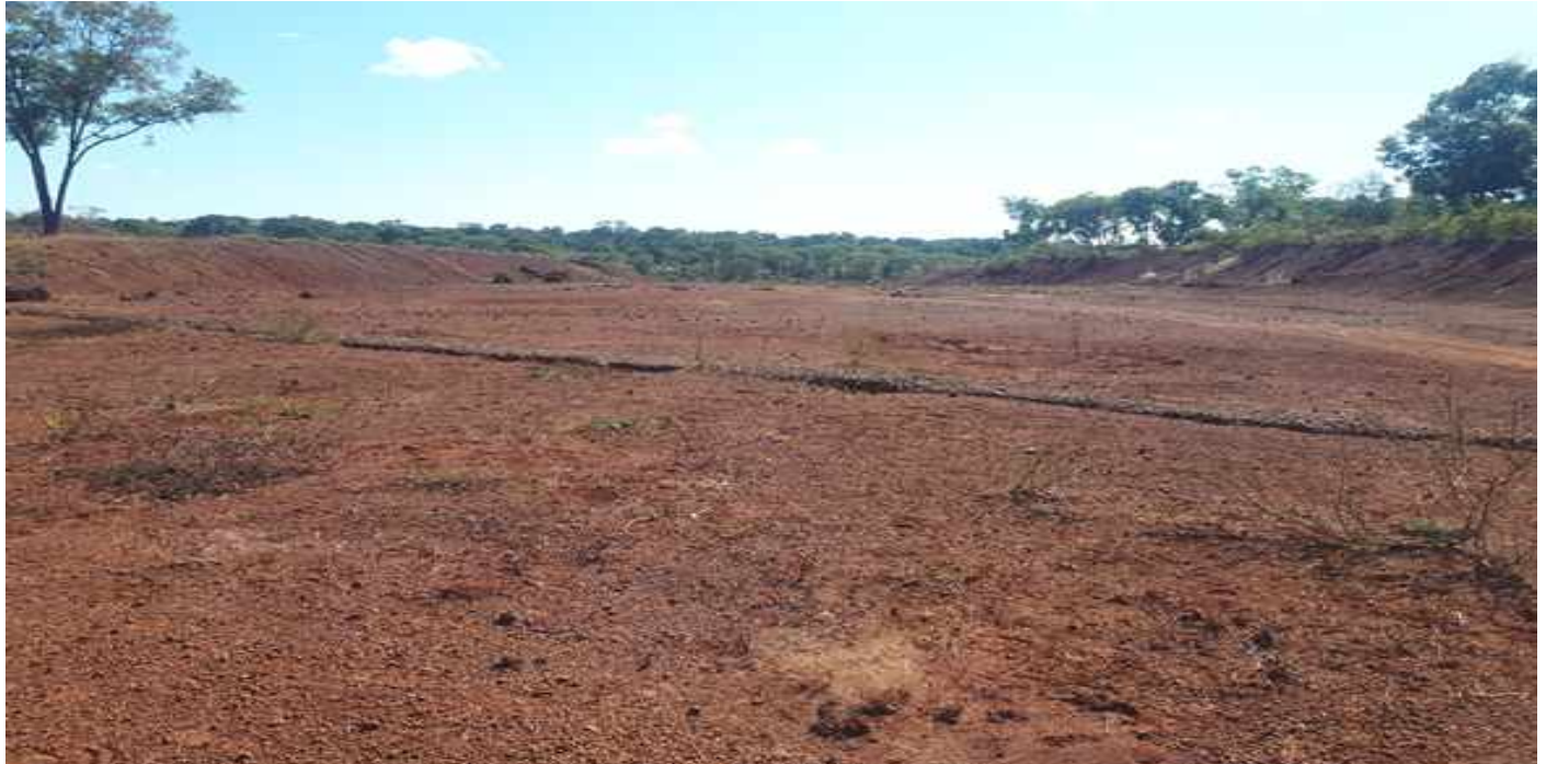
Plate 11: Spillway Return Channel Showing Straight Flow Path
