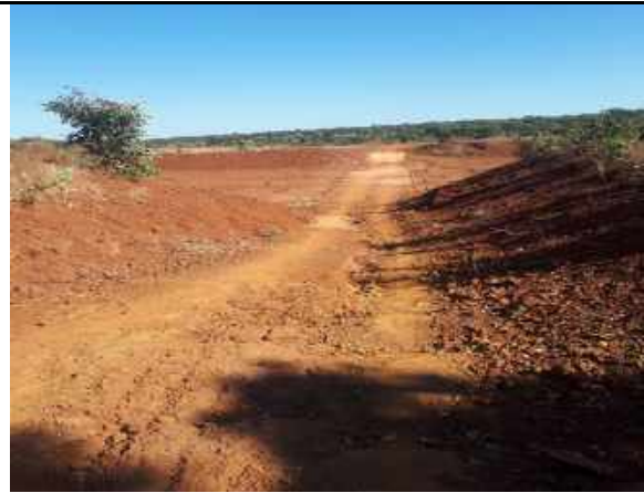
Access drift across the spillway channel
