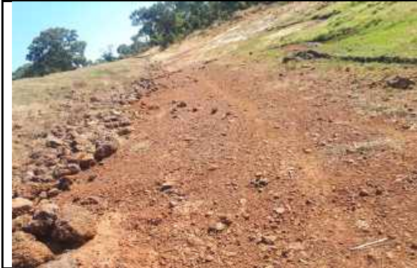
Damaged protection of the upstream berm
