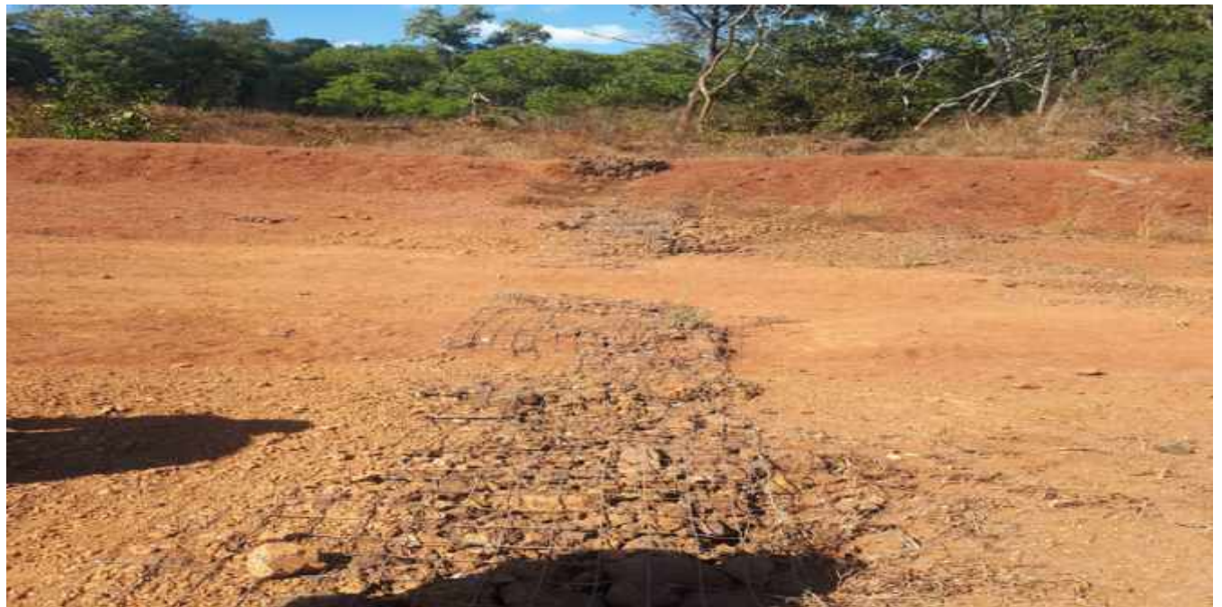
Plate 10: Damaged Spillway Gabion Sills
