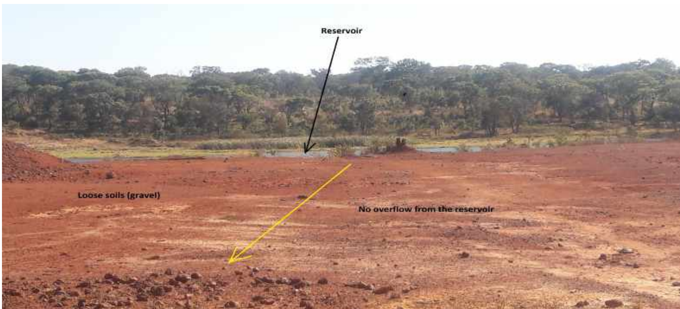
Figure 7: Portion of spillway completely dry. Surface unprotected from erosion
