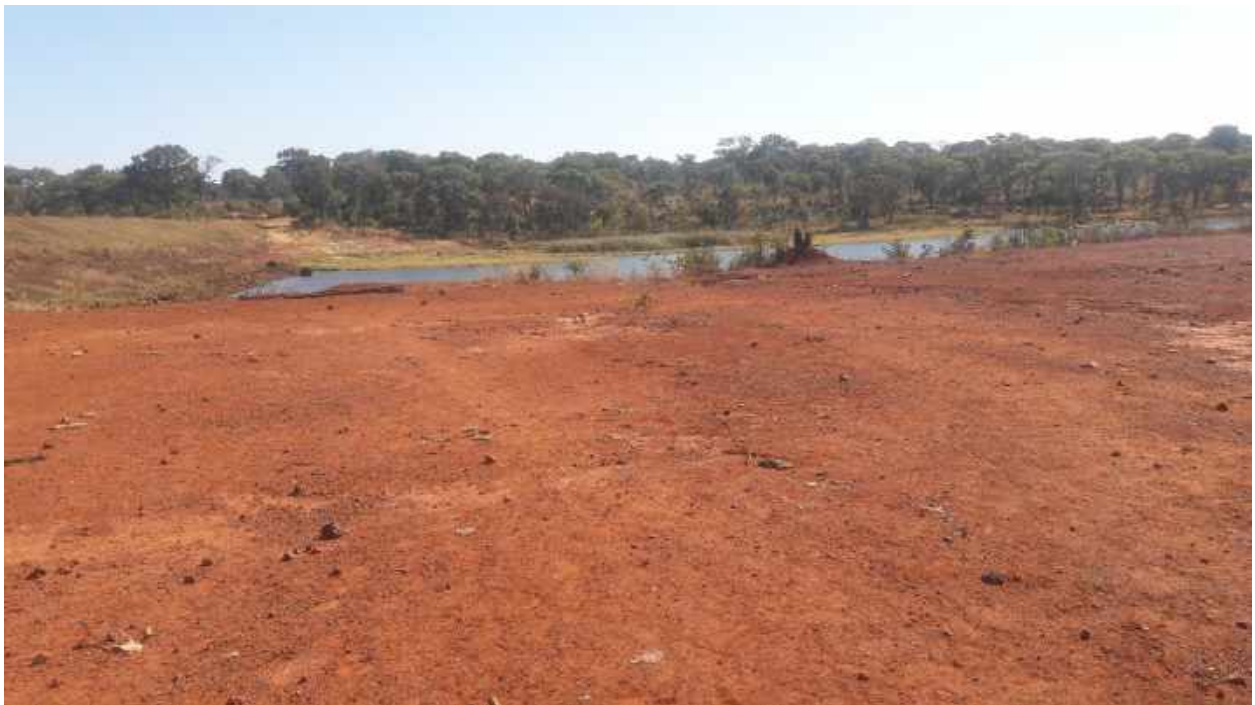
Plate 19: Spillway return channel needing rework to arrest erosion and sedimentation
