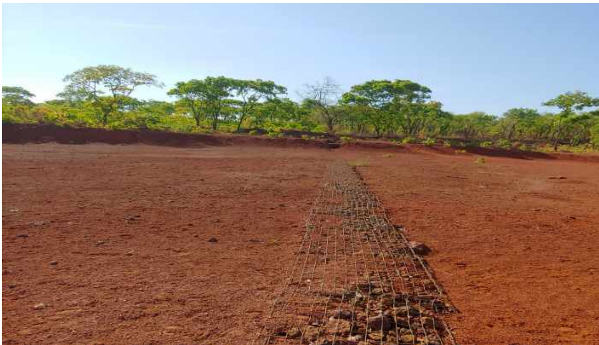
Plate 23: Gabion Basket Erosion Protection Structure
