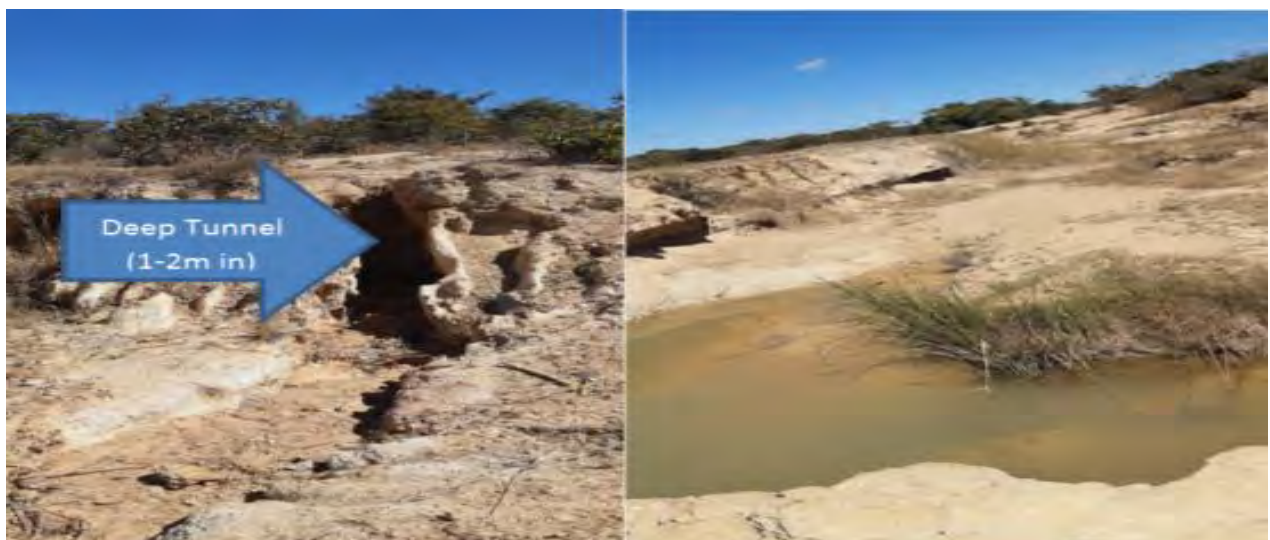
Figure 22: Gullying in the return channel
