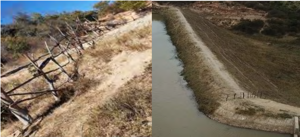
Figure 19: Fencing at left flank to avoid animal crossing over the embankment
