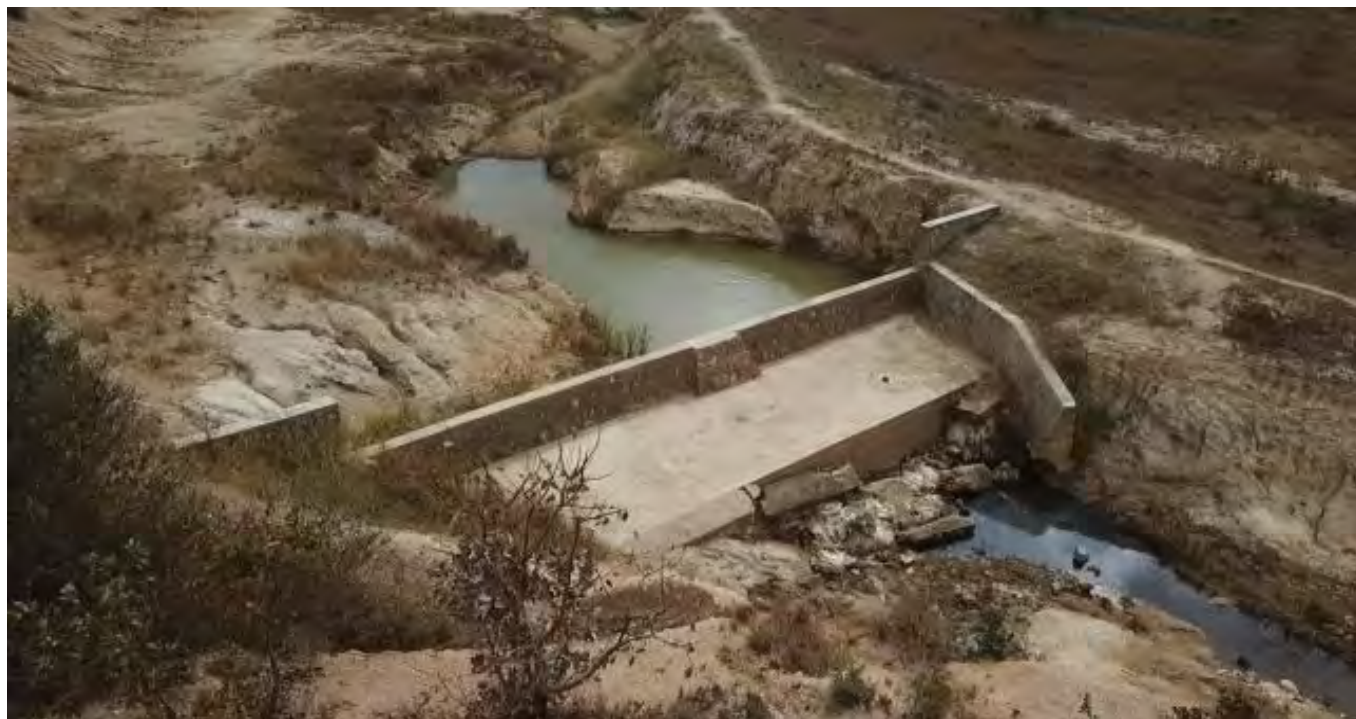
Drop structure flood damage since 2018.
