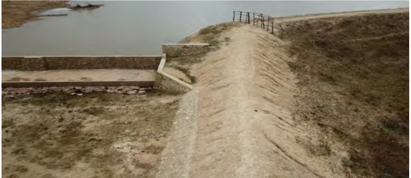
Gully erosion on external face of training wall
