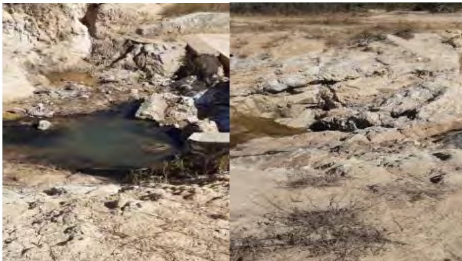
Figure 2: Deep eroded rock structures in the spillway bed
