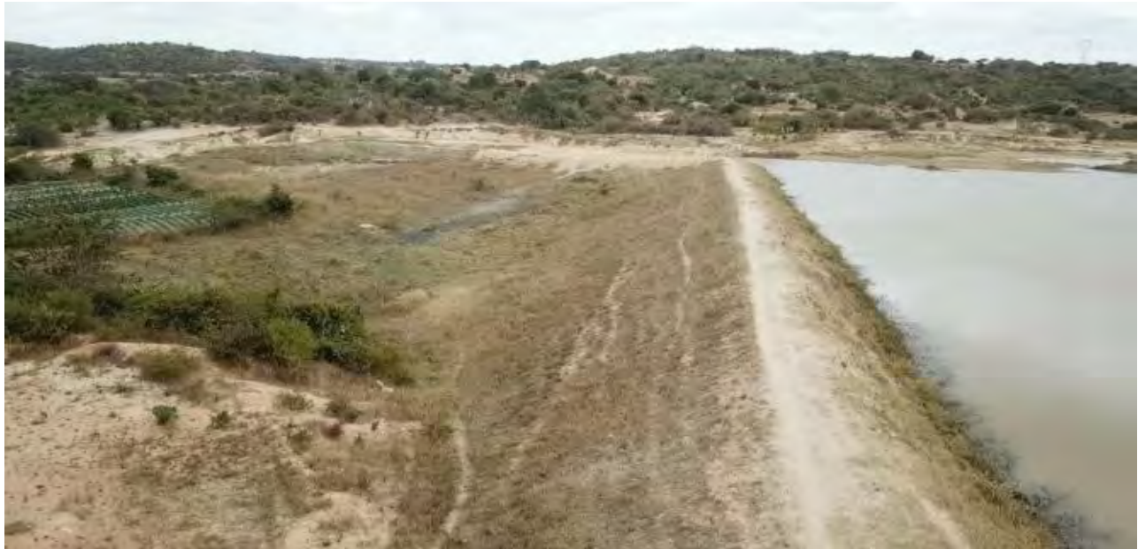
No evidence of toe drain or rock toe
