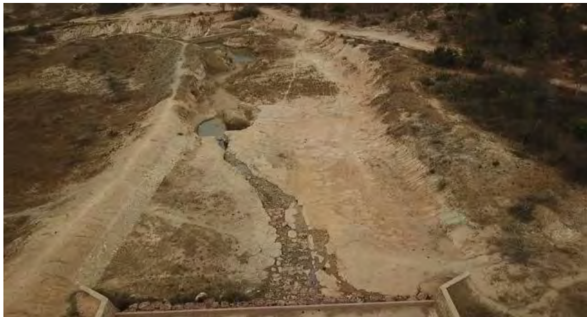
Aerial view of spillway return channel down to drop structure
