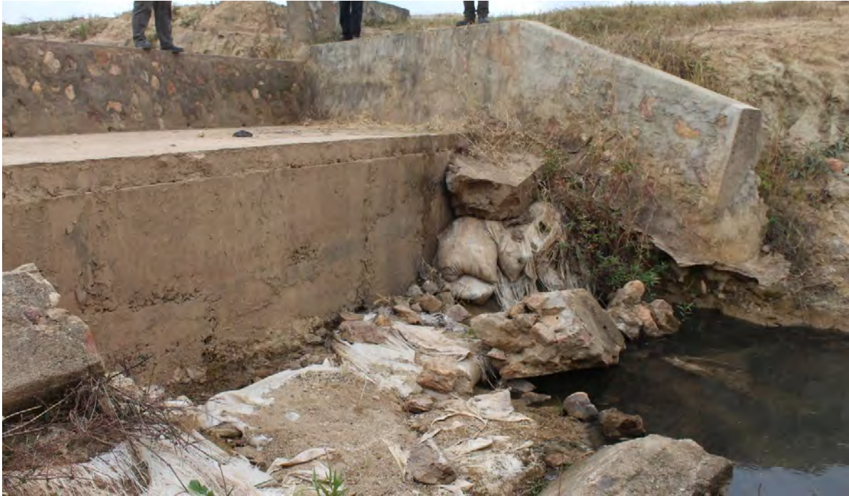
Figure 38: Drop structure showing undercutting of left hand abutment (to be removed)
