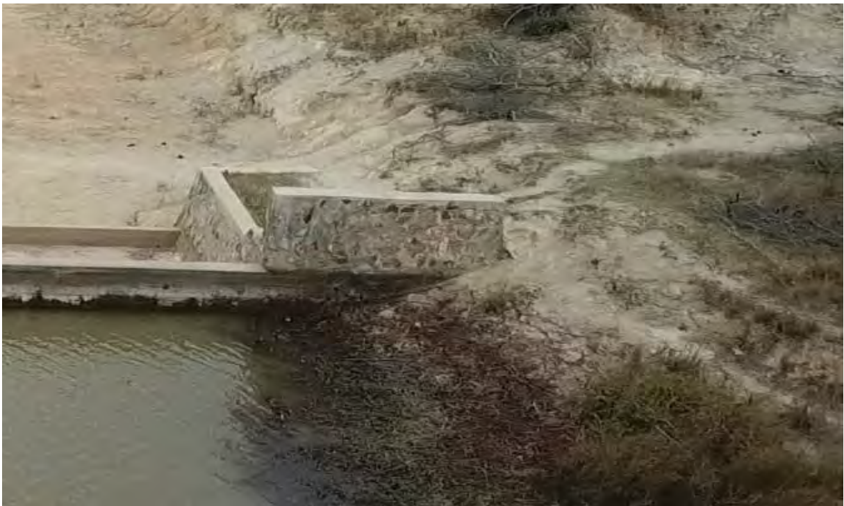
Figure 35: Right abutment potential for bypassing at higher floods
