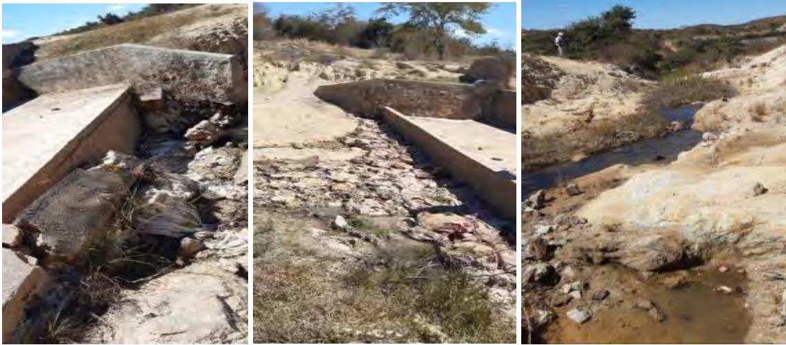
Figure 20: Spillway/ drop structures' state
