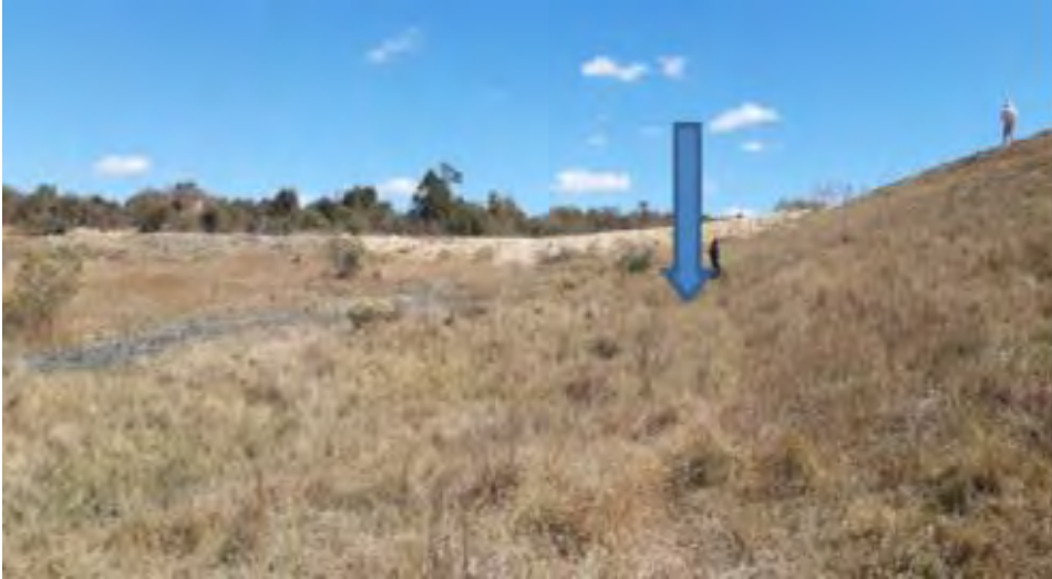
Figure 17: Seepage point towards right flank
