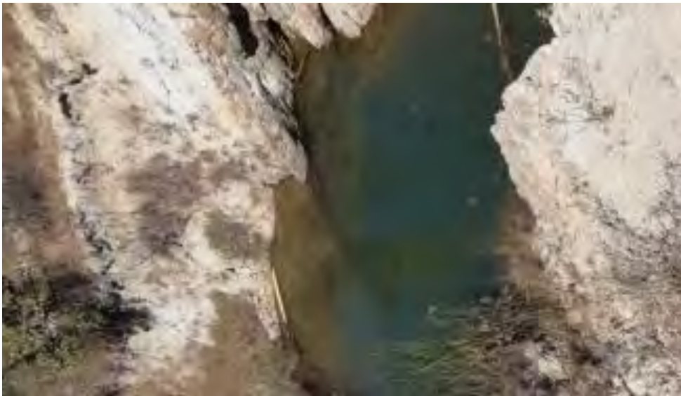
Figure 30: Depressions with stagnant water between drop structures
