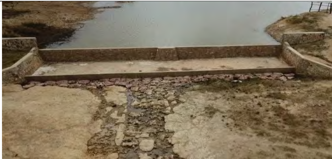
Spillway from downstream showing condition of sandbags from last season
