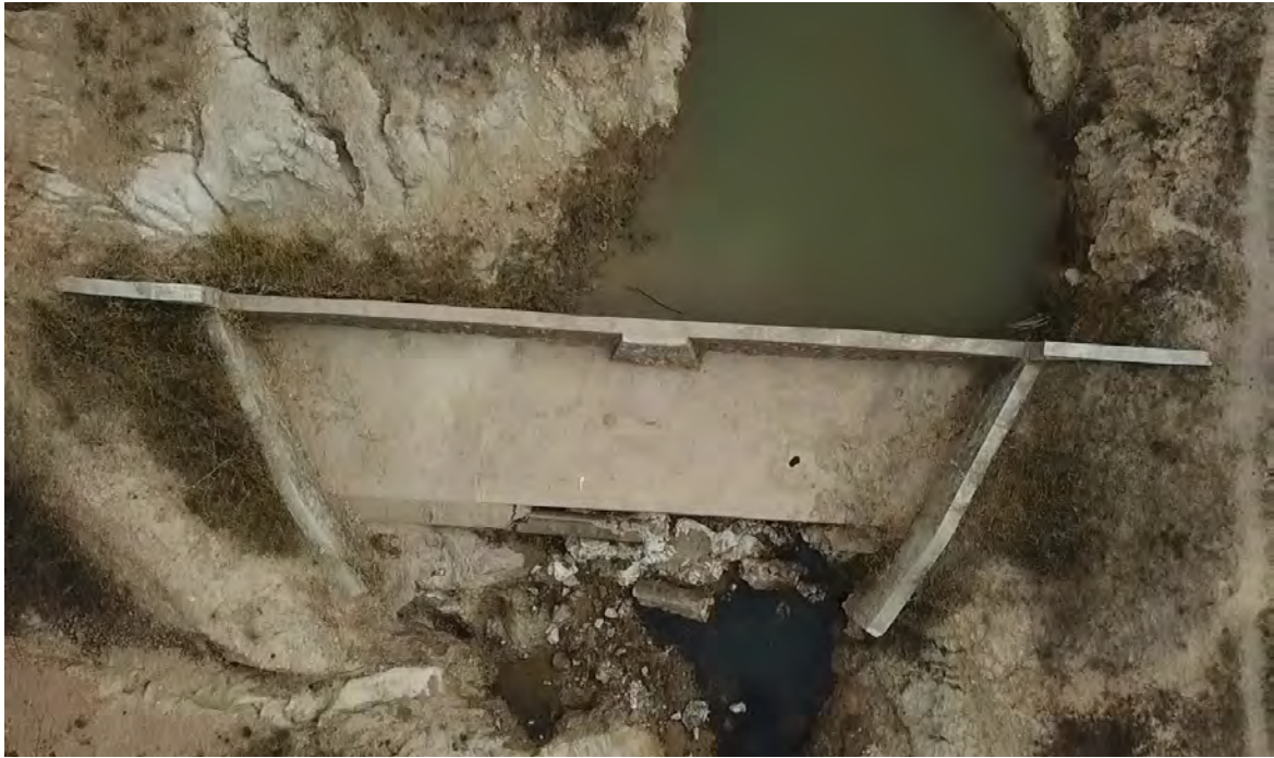
Figure 37: Drop structure upstream gulley and gabion repair locations
