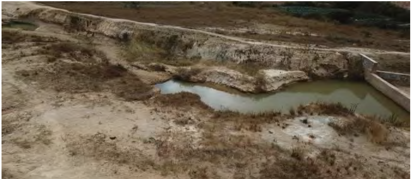
Spillway channel showing current state of training wall
