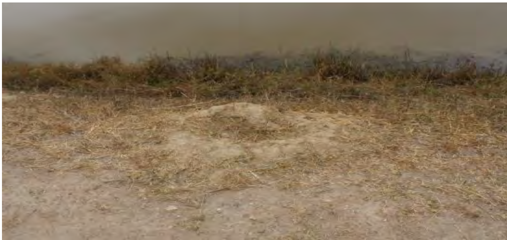
Figure 21: Termites workings on the crest edge and front face
